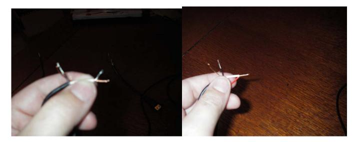
**Step 6:** Apply electrical tape around the twisted ends of the wires.
